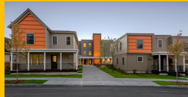
Photo source: Duncan Wisniewski Architecture
